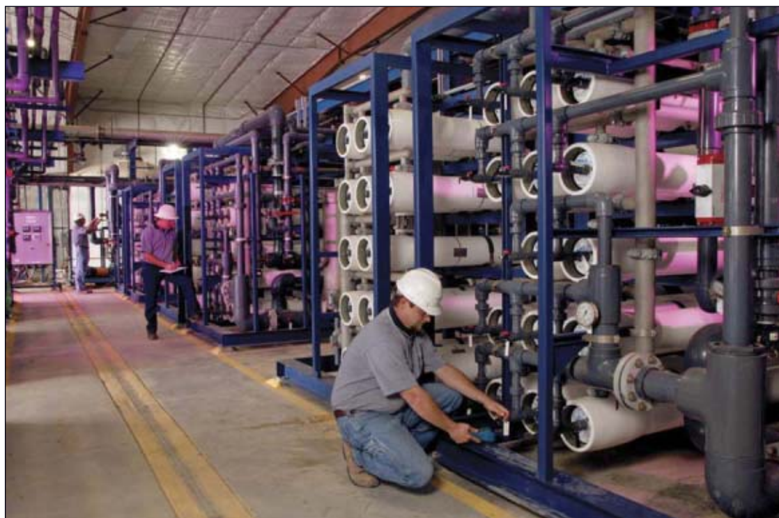
The Wild Turkey plant RO-based treatment system prepares the water for surface discharge (Fig. 3).
