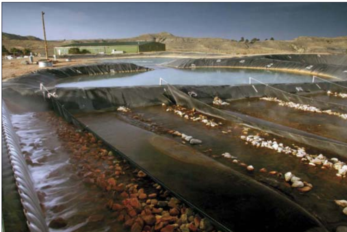
The produced water stream enters a ballast pond before being pumped to the Wild Turkey treatment facility (Fig. 1).
